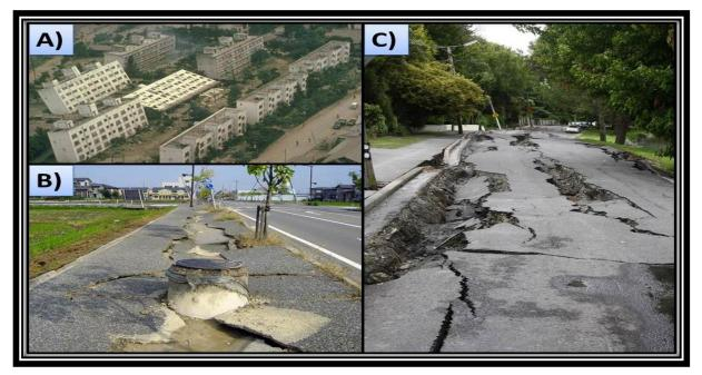
Figure 38: Example of soil liquefaction
