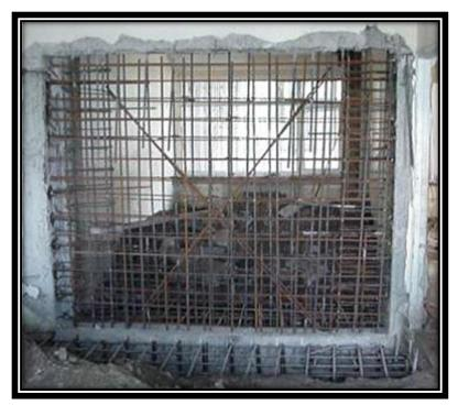
Figure 83: Additional Shear Wall
