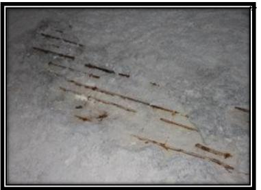
The climatic conditions of an area have a great influence on the corrosion rate. In extreme climatic conditions in coastal regions, the rate of corrosion will be high. For example, the Gulf Coast has an extremely aggressive environment, characterized by high ambient temperature humidity and
